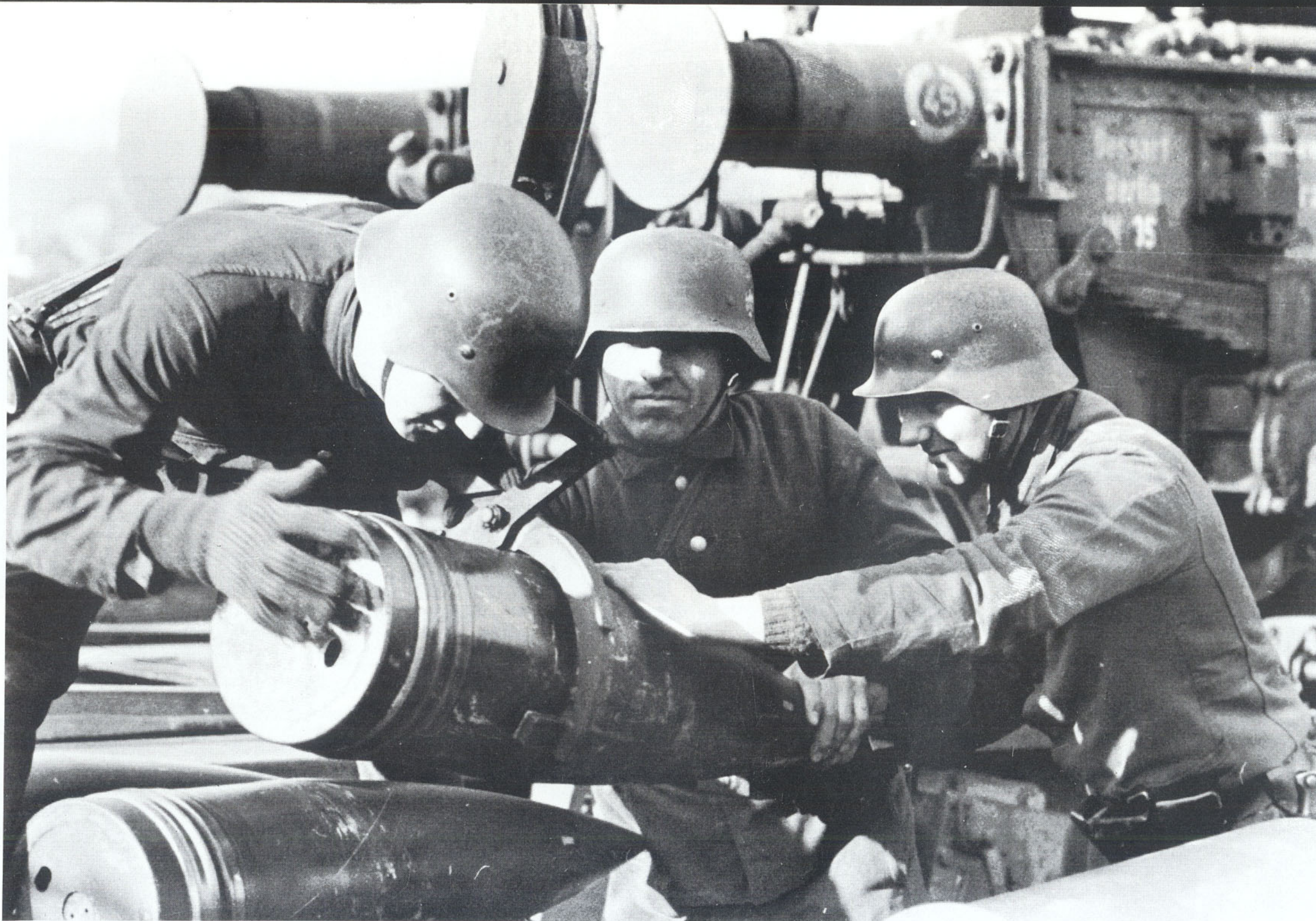
The loaders have placed a shell into the clamp of the loading crane, and it will then be lifted up to the loading cradle behind the breech. Note the rotating bands on the projectiles. These engaged the rifling in the barrel to rotate the shell to stabilize it, and also to form an effective gas seal for the best range.
