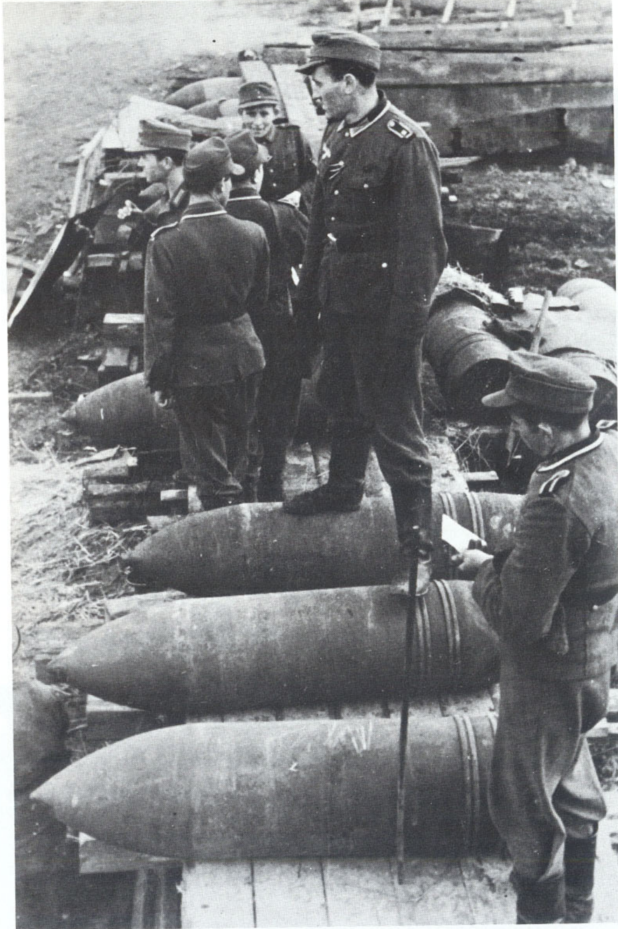
These shells for the 37 cm French railroad gun—seen on the previous page—were about 1.60 meters long, and have been laid out along this planked deck so that they can be rolled up to the gun as quickly as the crew can fire and reload.
